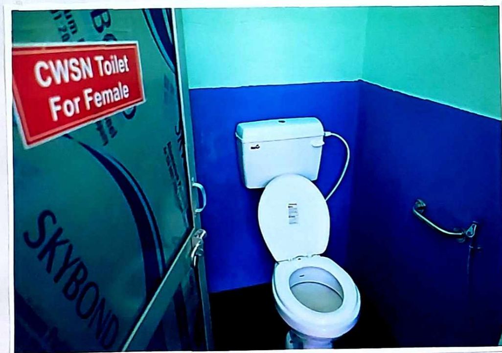
GROUND FLOOR CWSN TOILET FOR FEMALE
